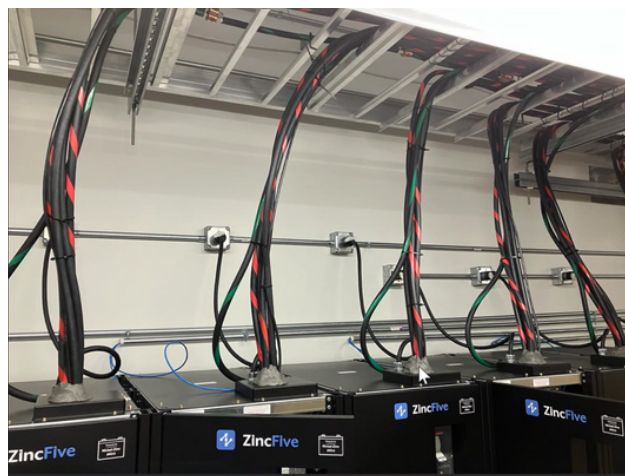
Figure 8 - Field example of standard wire installation
